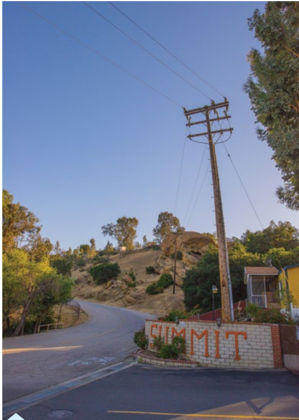
POWER TOWER: SCE power pole looms over Summit entrance. Electricity is transmitted at high voltage over the poles until it reaches apartments and housing tracts where it is stepped-down to serve the 120-volt power needs of toasters and television sets. Larry LaCom/Summit Life photo.
